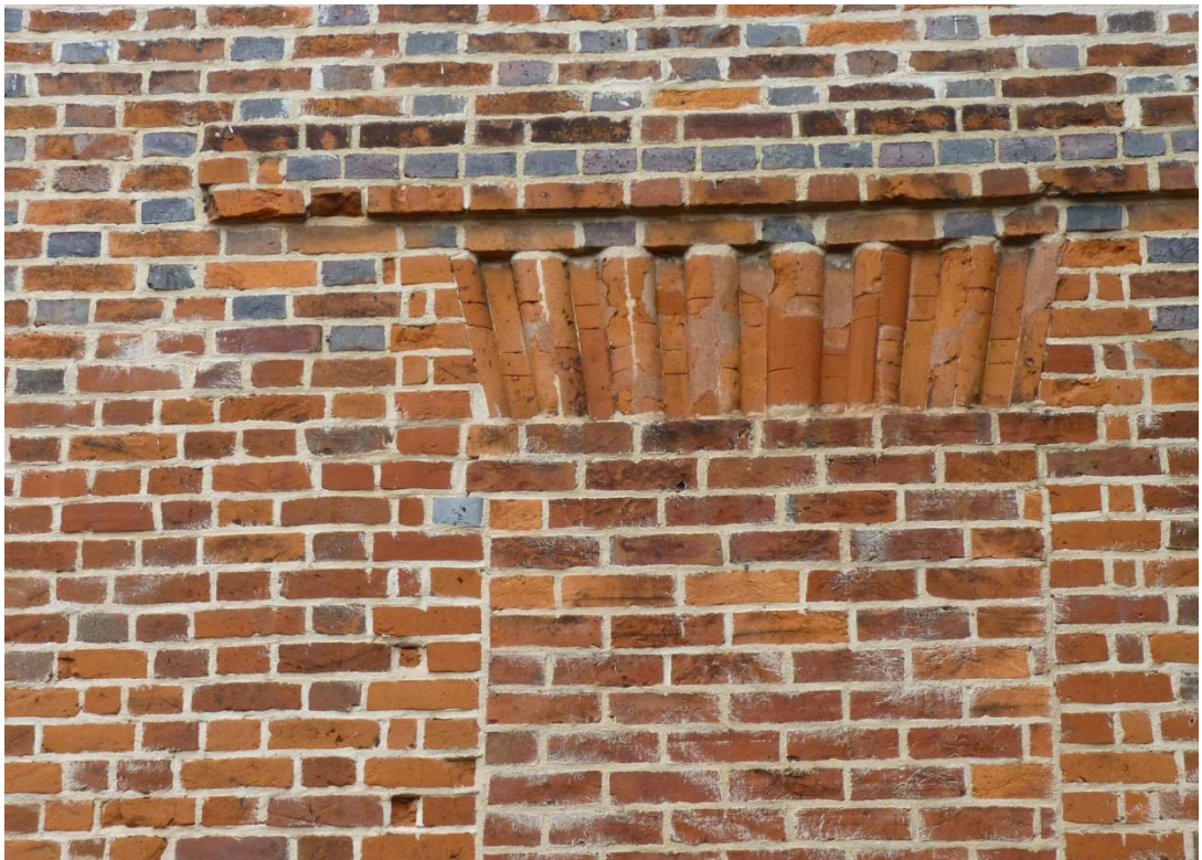
Contrast of brick coursing/poor mortar repairs – High Street
