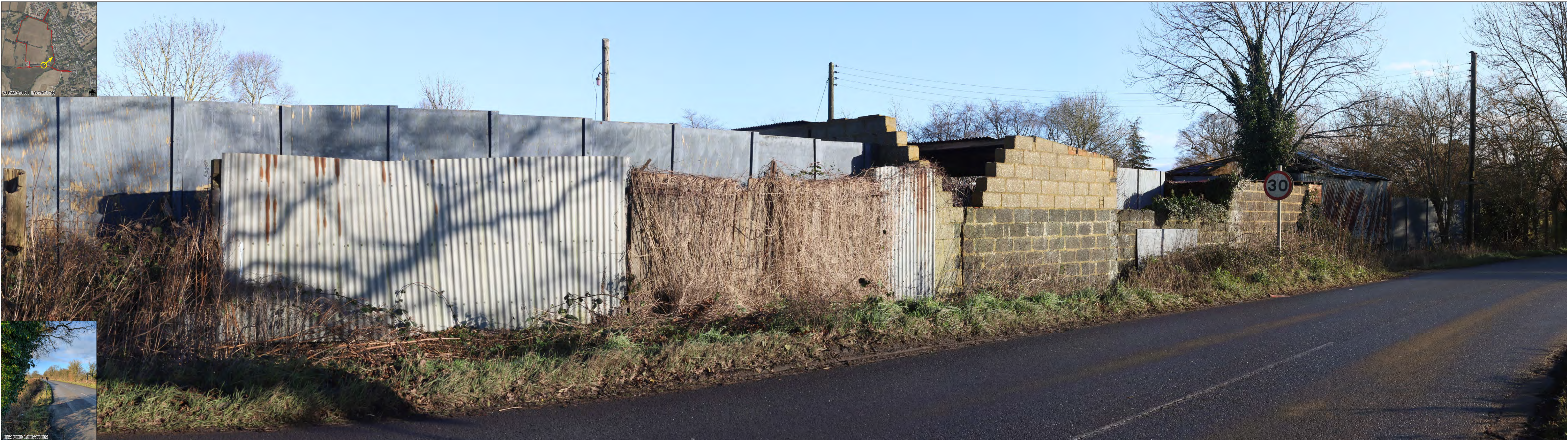
EXISTING BASELINE VIEW
