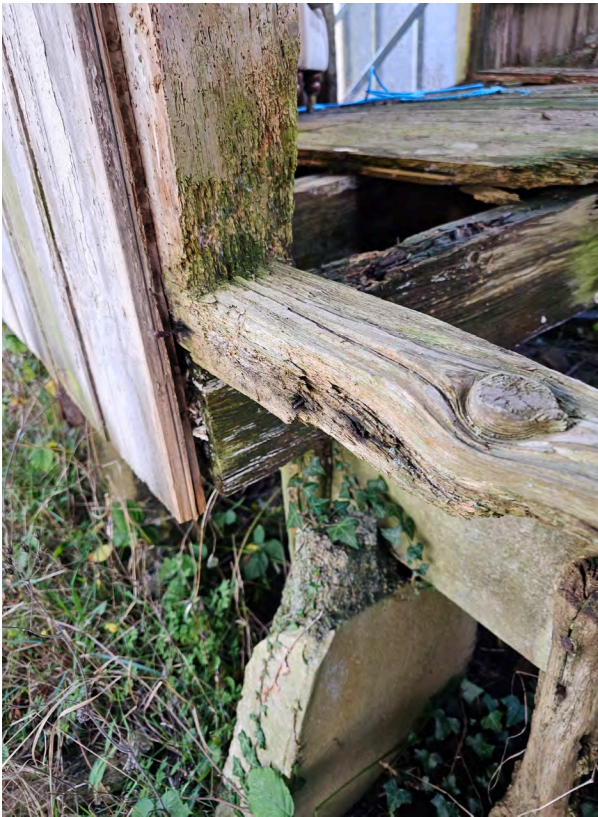
cill plate, door post, joists and cladding
