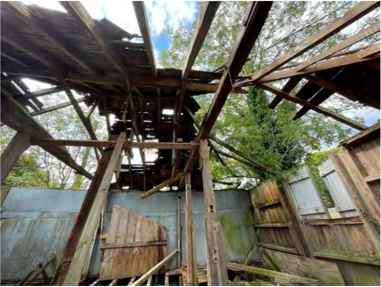
internal face of south elevation showing central posts
