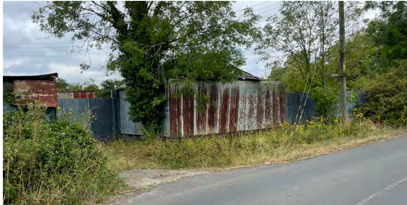
south elevation from road
