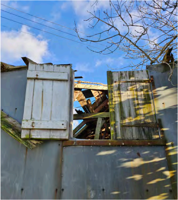
external face of shutters to west elevation
