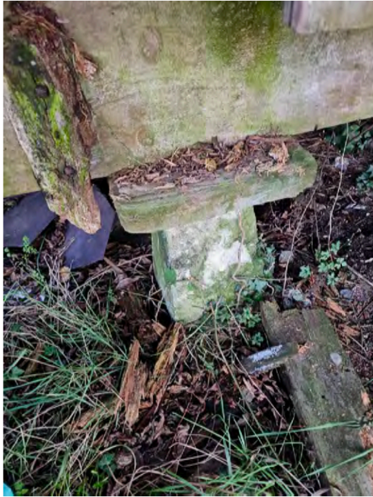
staddle stone supporting girder
