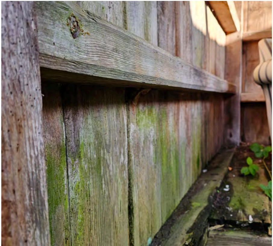
rail and cladding
