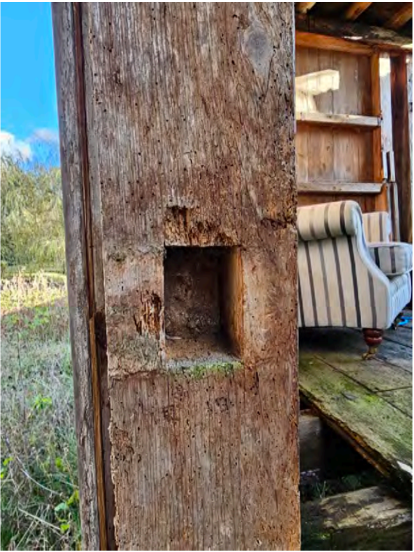
mortice in post to receive cladding rails
