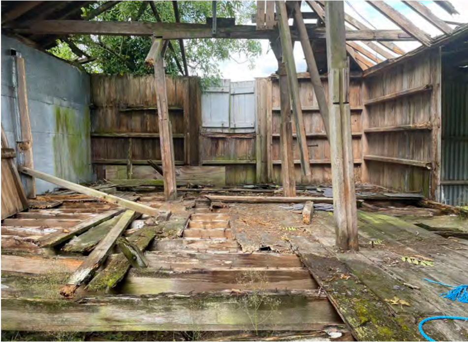
internal face of west elevation
