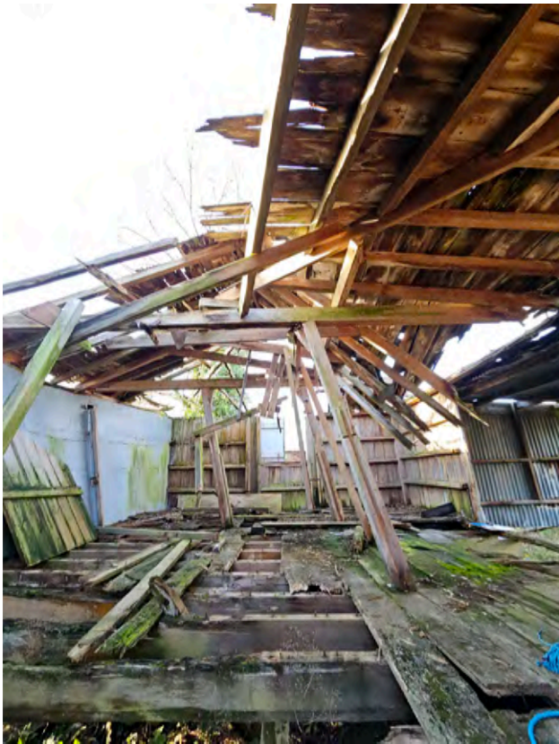
tie beam morticed and pegged to posts
