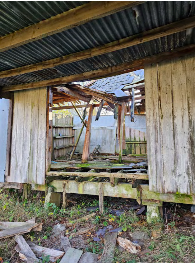
opening and original external cladding to north elevation
