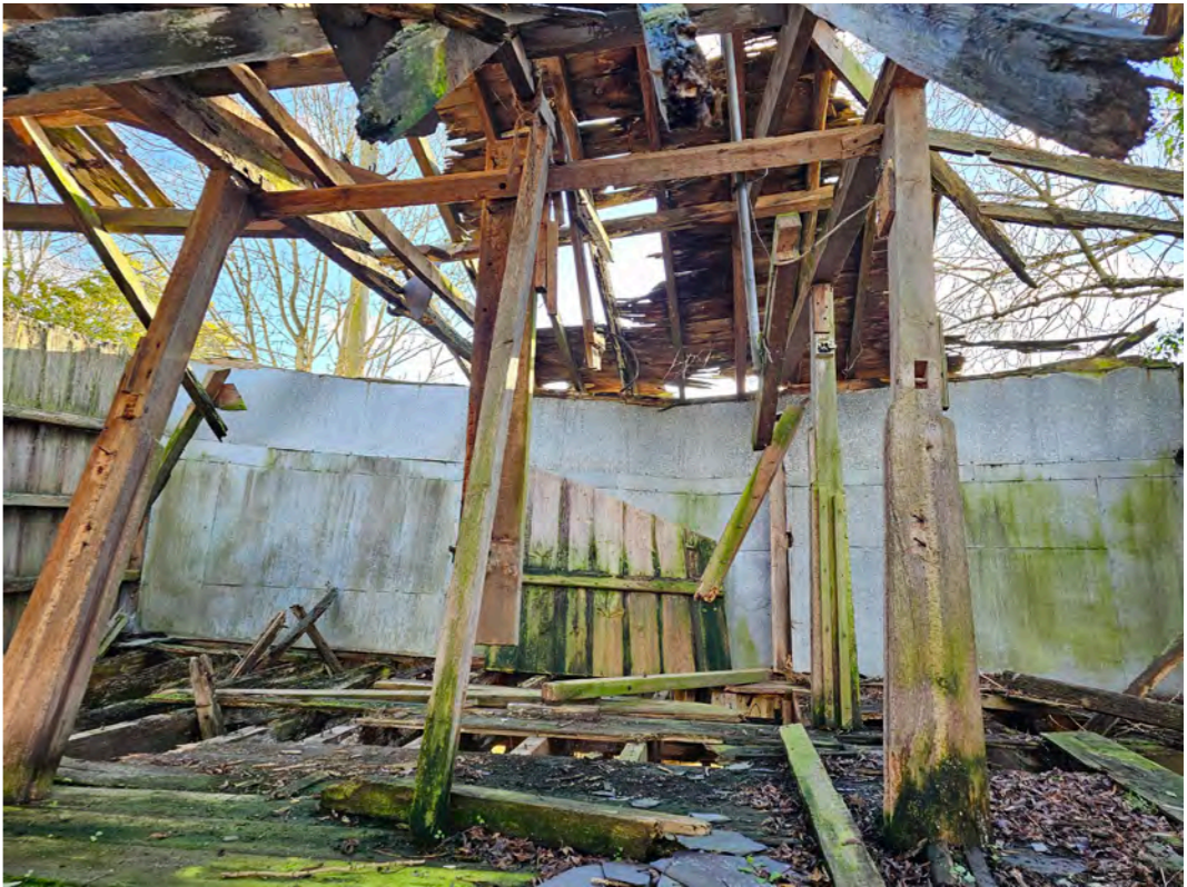
haunched central posts to grain bins. Note pegs and mortice to receive partitions (re- mant of partition propped on rear wall)
