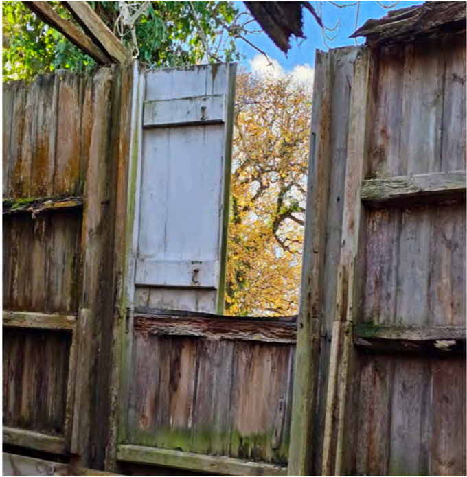
internal face of shutters to west elevation
