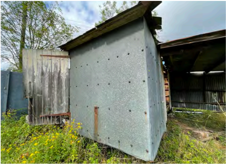
external face of door to east elevation
