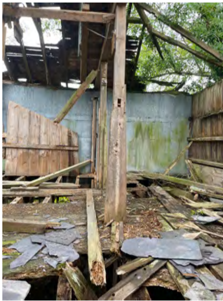
mortice and peg in grain bin post to receive partition and remnant of grain bin partition
