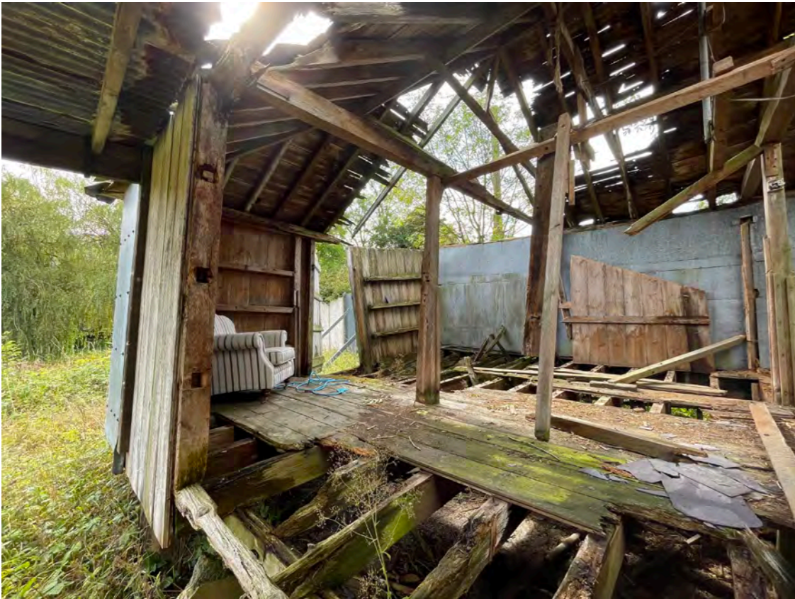
internal view of roof structure
