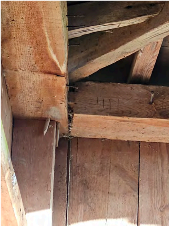
morticed and pegged wall plate and post
