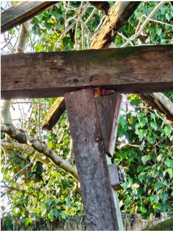
morticed and pegged post to tie beam
