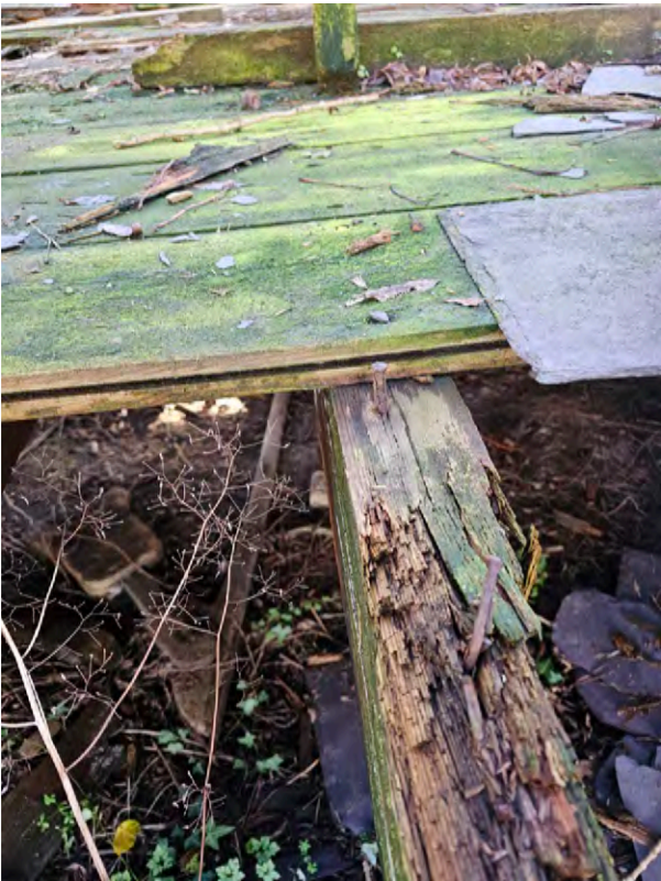
nailed tongue and grooved floor boards
