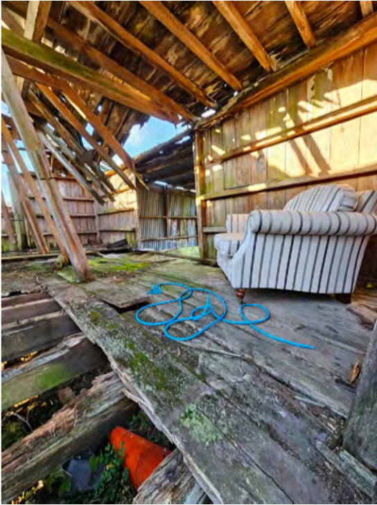
internal face of north elevation showing opening
