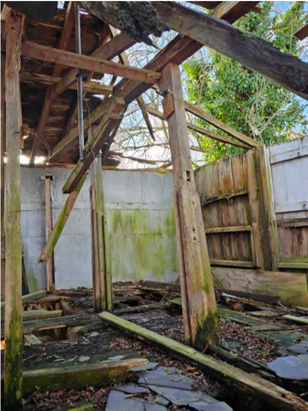
haunched and grooved central grain bin post supporting tie beam. NB brackets to be removed
