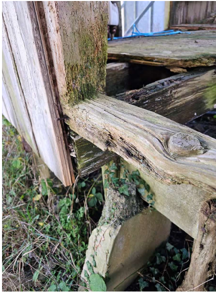
cill plate, door post, joists and cladding
