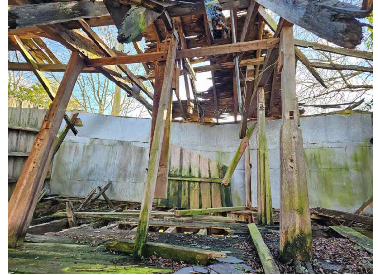
haunched central posts to grain bins. Note pegs and mortice to receive partitions (re- mant of partition propped on rear wall)
