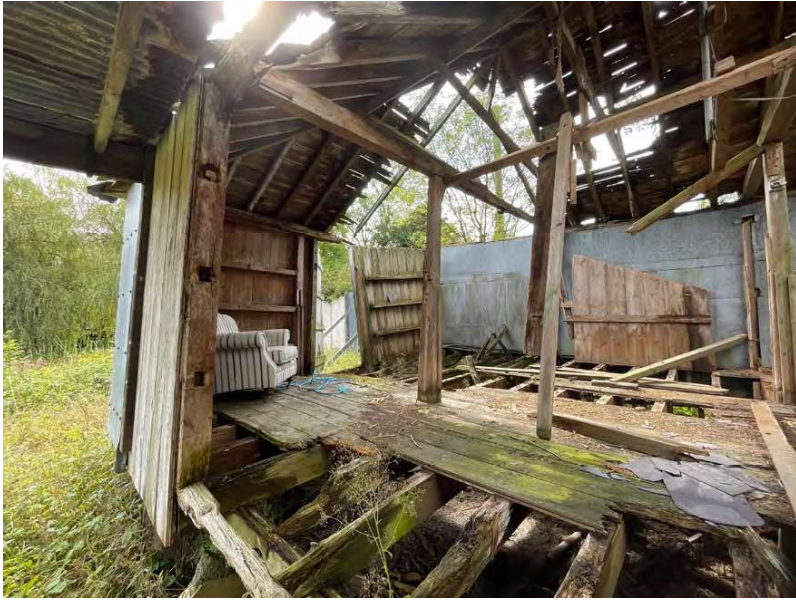
internal view of roof structure
