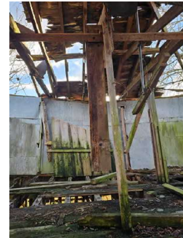
central grain bin prop supporting tie plate to be removed
