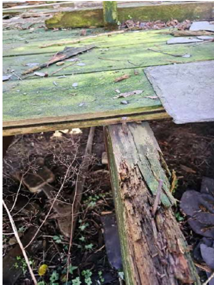
nailed tongue and grooved floor boards
