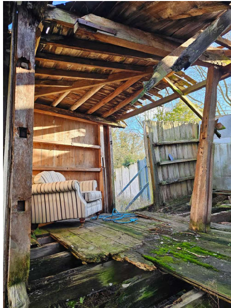
internal face of east elevation
