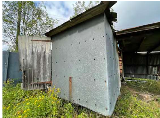
external face of door to east elevation
