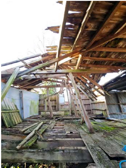
tie beam morticed and pegged to posts
