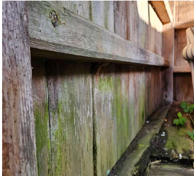
rail and cladding
