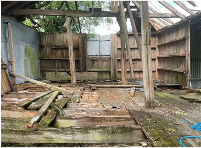
internal face of west elevation
