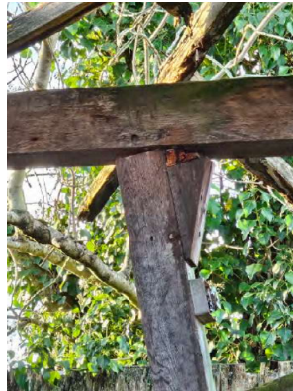
morticed and pegged post to tie beam
