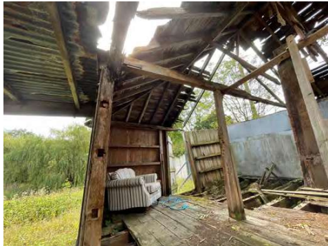
morticed and pegged wall plate and post
