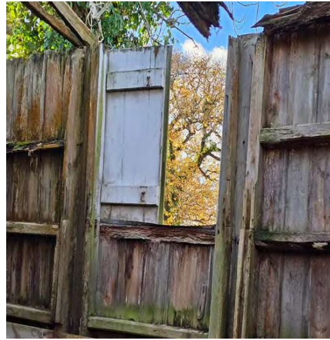
internal face of shutters to west elevation
