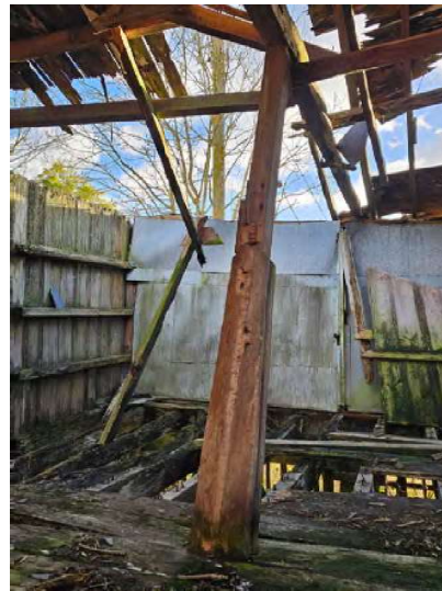
haunched and grooved central grain bin post supporting tie beam
