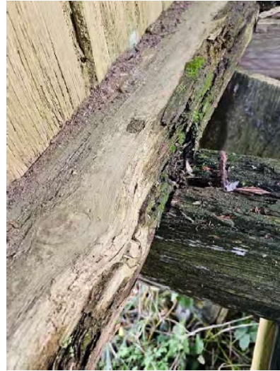
cill plate pegged (alternate) and lapped over joists
