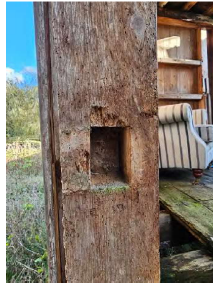
mortise in post to receive cladding rails
