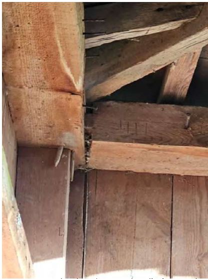
morticed and pegged wall plate and post
