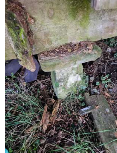
saddle stone supporting girder
