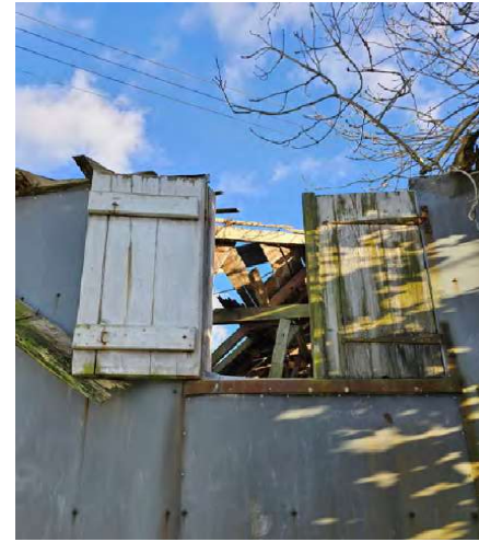
external face of shutters to west elevation
