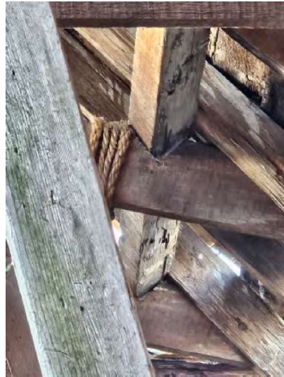
trenched purlin over collar (rafter appears lapped) Collar may be later
