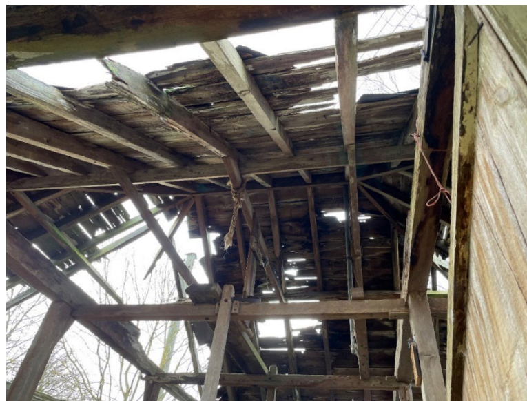
Plate 18: Structure A, detail of roof structure.
