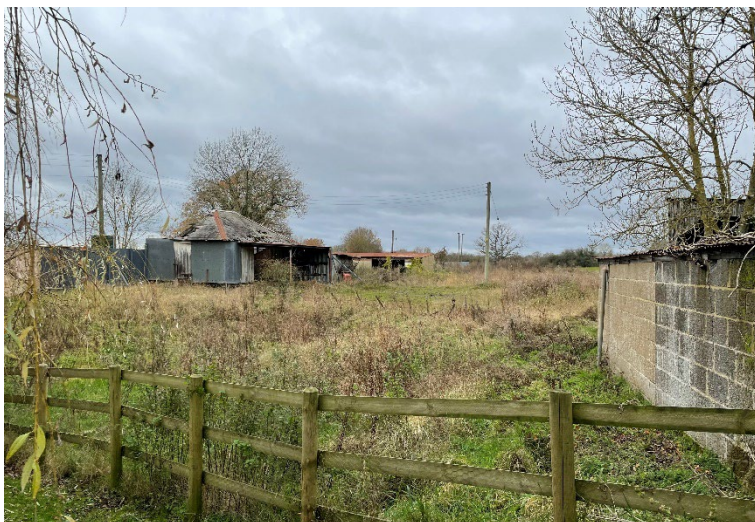
Plate 30: Views from The Moat Boundary towards Farm Building.
