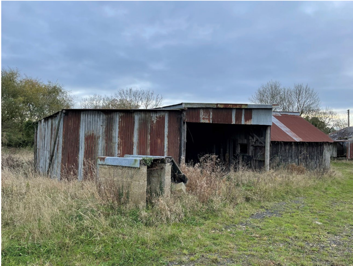
Plate 21: Structure E, general view of west elevation.
