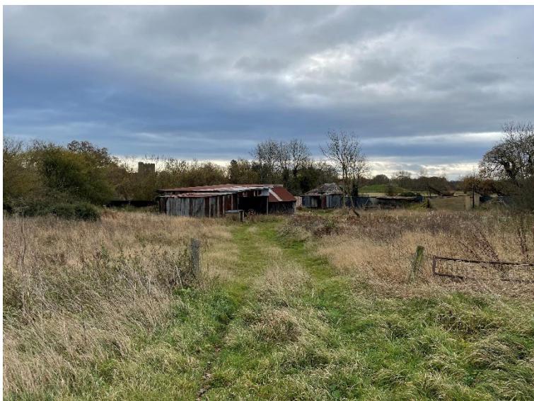
Plate 28: Views South Towards the Farm Buildings from the Site.
