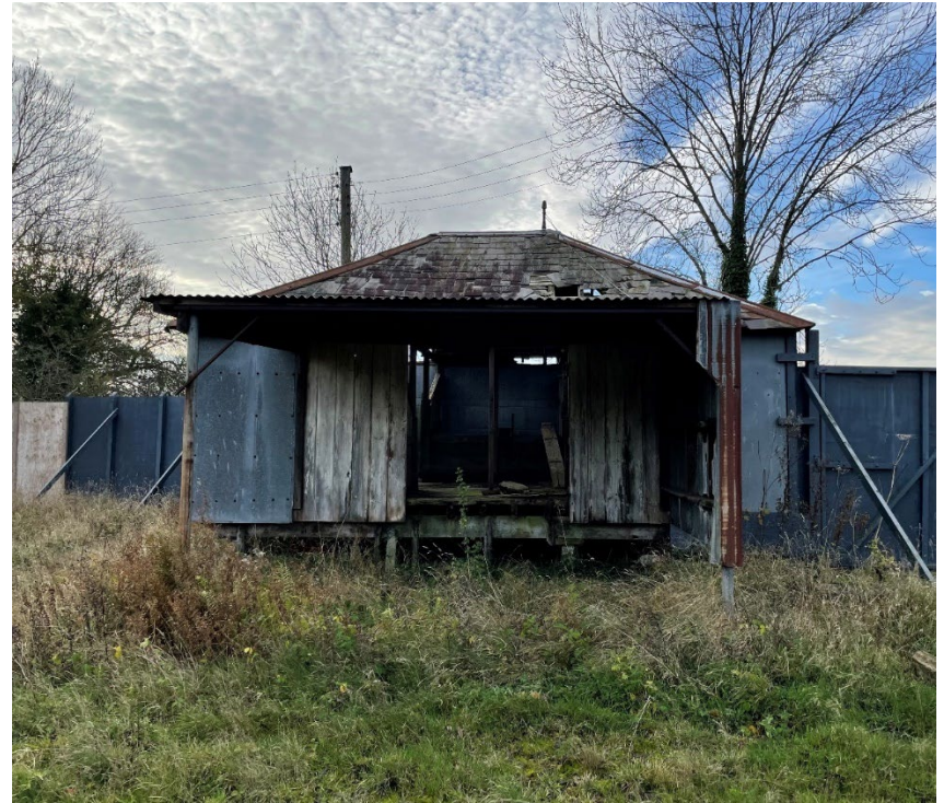
Plate 16: Structure A, general view of north elevation.
