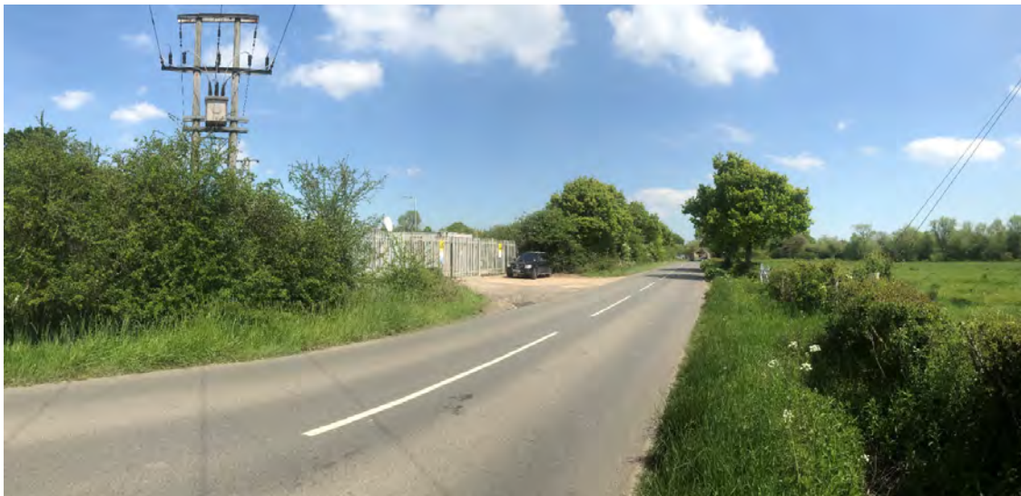
Image EDP 2.3: Looking along Moat Road, from the west, towards the substation and proposed site access point.
