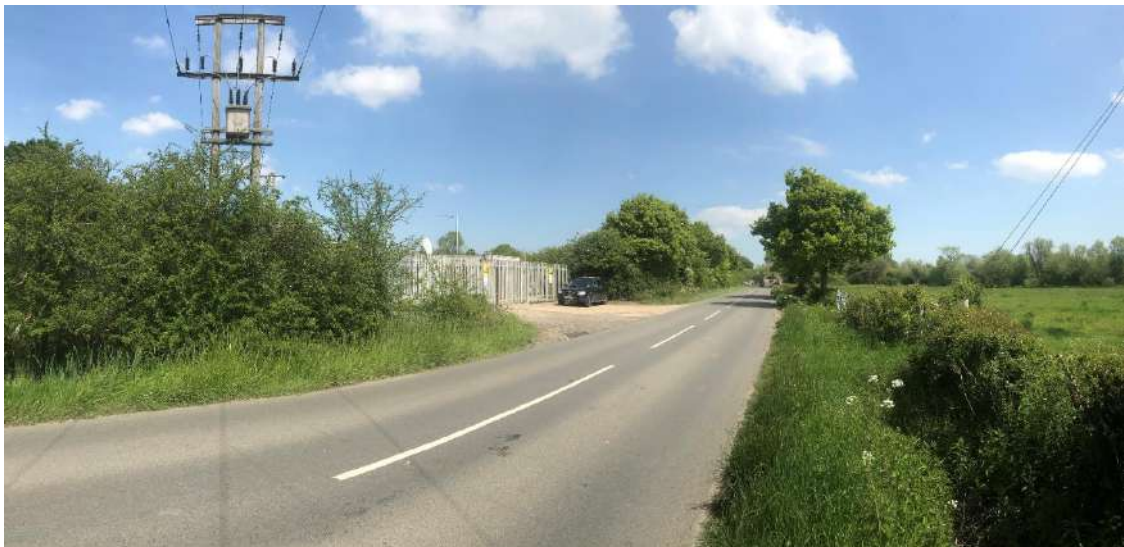
Image EDP 2.3: Looking along Moat Road, from the west, towards the substation and proposed site access point.
