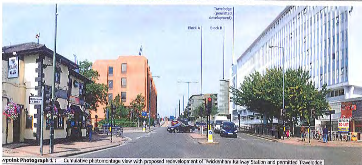
Photograph 1: View north from pedestrian crossing at junction of Arragon Road and London Road (September 2010)
