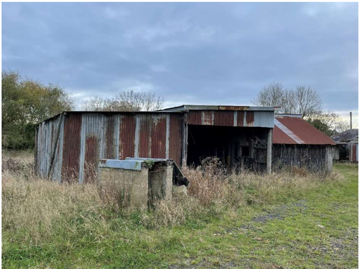
Plate 12: Structure E, general view of west elevation.
