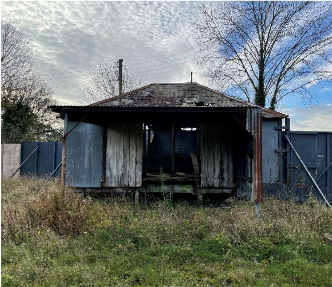
Plate 7: Structure A, general view of north elevation.
