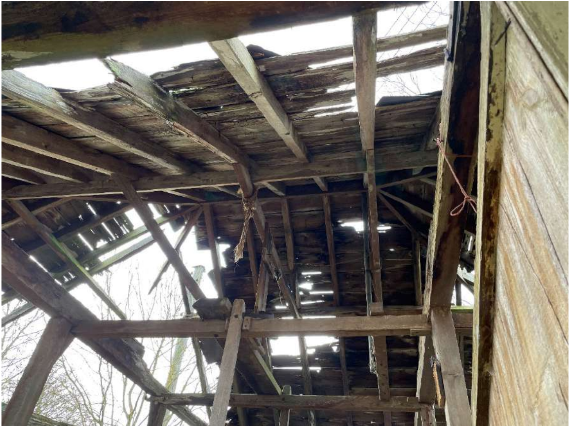
Plate 9: Structure A, detail of roof structure.
