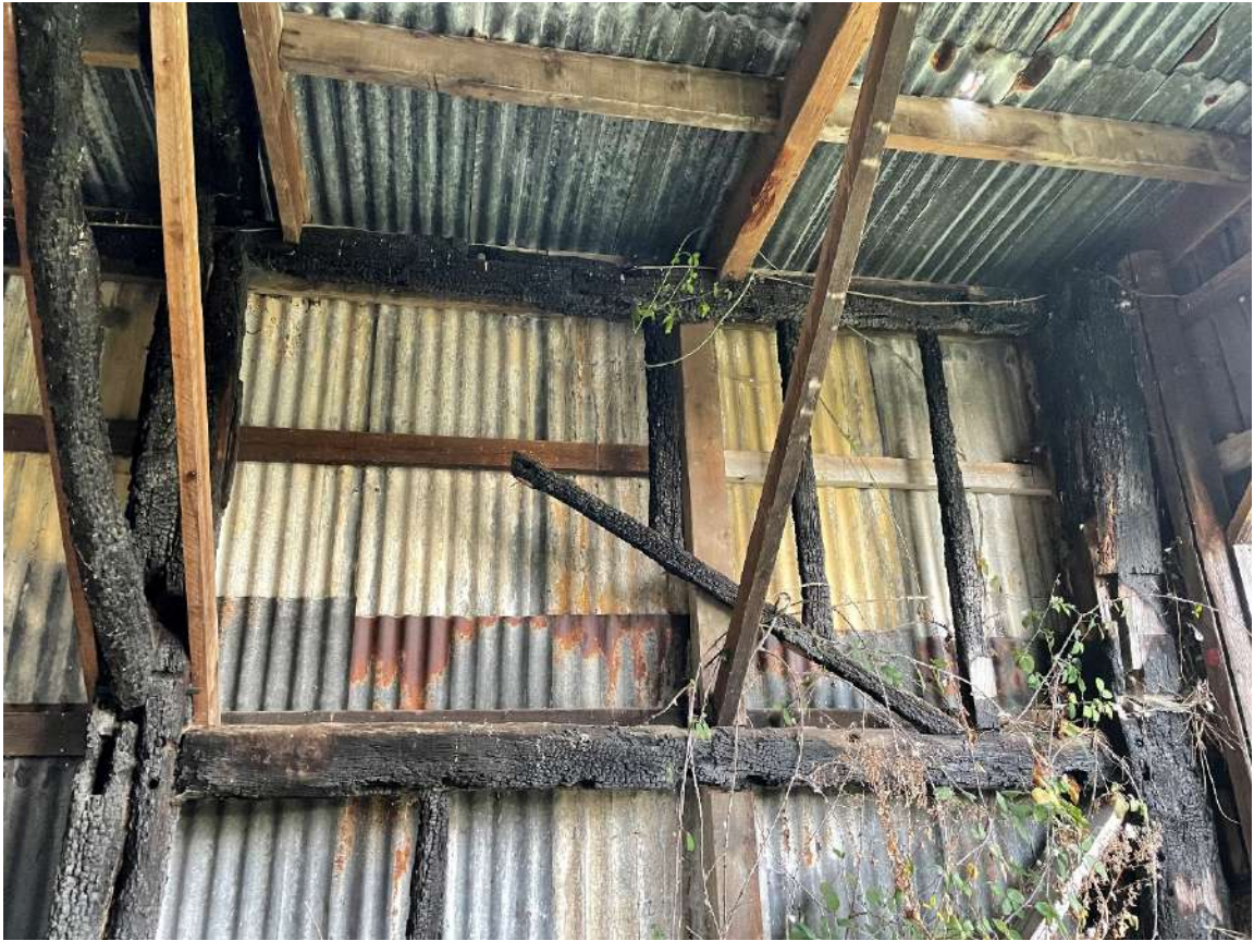
Plate 13: Structure E, detail of interior.
