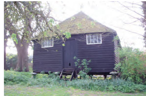
Detached granaries of this type, raised on mushroom-shaped staddle stones, are found across the arable-farming vales and downlands of the AONB.
