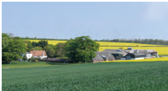
Large-scale loose courtyard farmstead, East Kent Downs (Area 10). These large farmsteads are typically marked by one or more large barns and a farmhouse of 17th century or earlier date, the granary, stabling and cattle housing built around the yard being much lower in profile.
