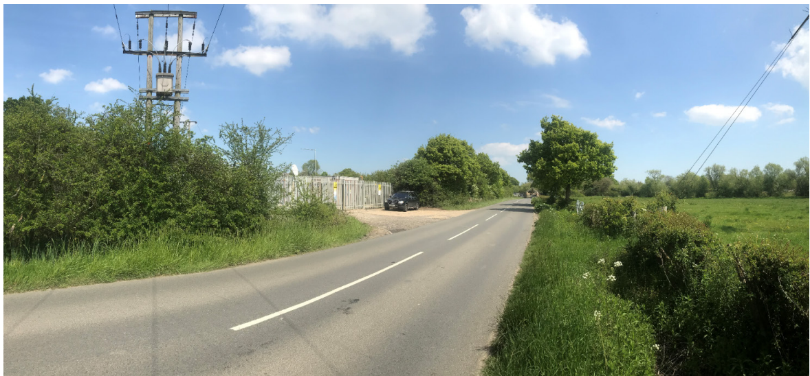
Image EDP 4.3: Looking along Moat Road, from the west, towards the substation and proposed site access point.
