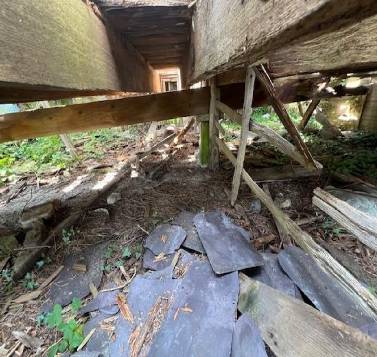
The photo here shows the underside of the timber joists.
