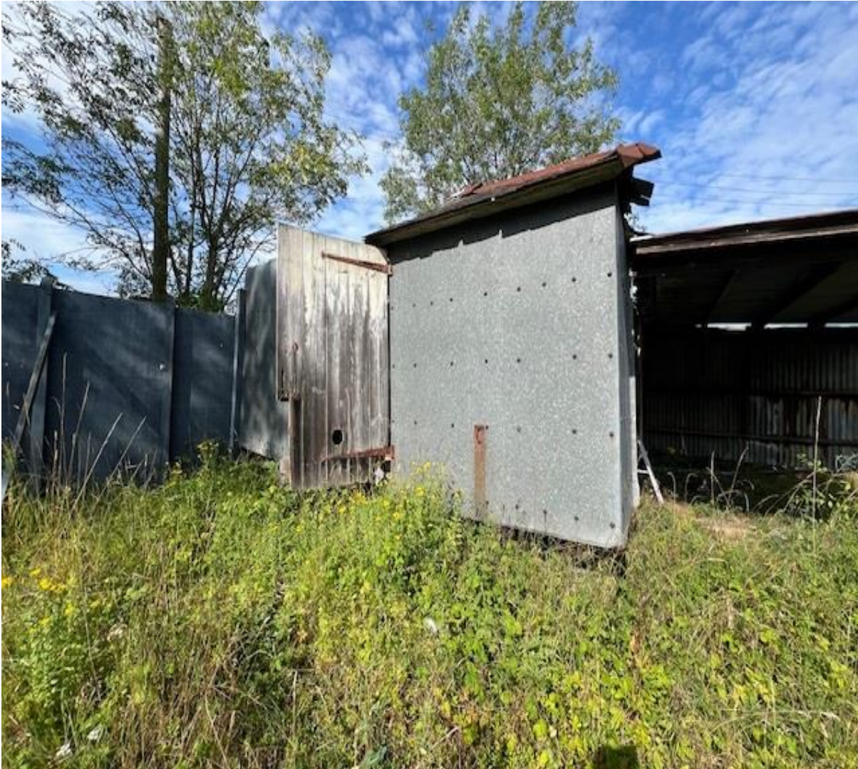
Metal cladding that sits at the external of the building
