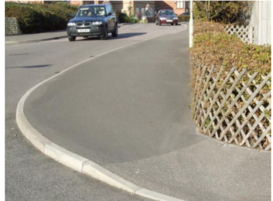
False widening' of footway to meet junction visibility requirement.
