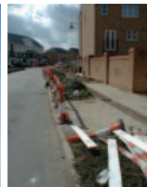
Above, where existing paving is disturbed to allow for the installation of services it should be reinstated with the original or closely matching materials, particularly in the case of traditional brick, stone, stone setts and cobblestone pavings.
