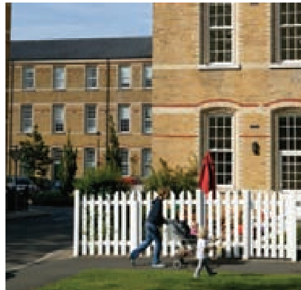
Reuse of buildings is sustainable and can lend a character that raises values in new development. (Caterham Barracks, by Linden Homes)
