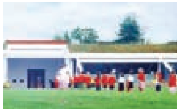
Minimising impact on-site This school keeps energy consumption to a minimum by hugging the contours of the site and maximising solar gain (Riverhead School, Sevenoaks, KCC)
