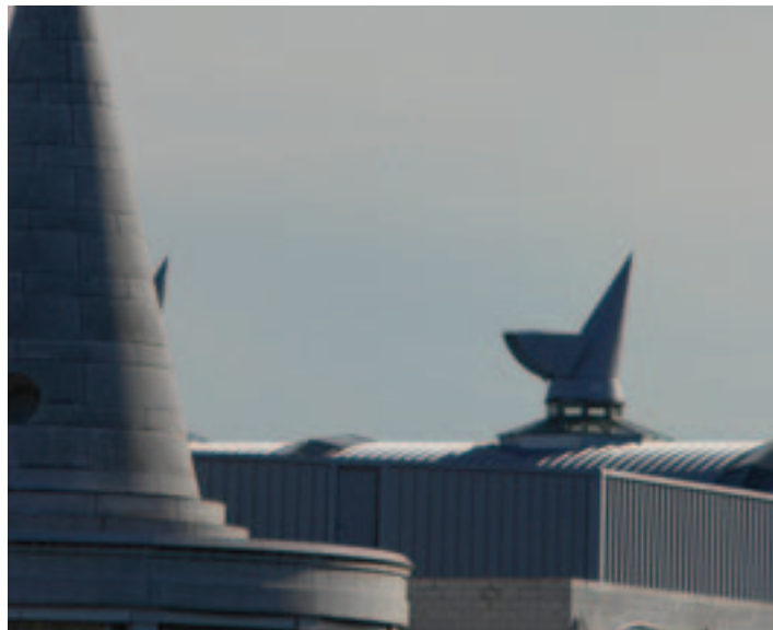
At Bluewater , building services create a distinctive silhouette inspired by the classic Kentish oast house coving. (Lend Lease)
