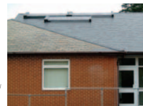
Historically, Kent residents and businesses have used the earth's natural resources to provide energy efficiently. Bottom, Swadelands Comprehensive school in Lenham was the first secondary school in Kent to receive eco-school status in 2001. They have installed a solar thermal space heating system with the help of Creative Environmental Networks (CEN).
