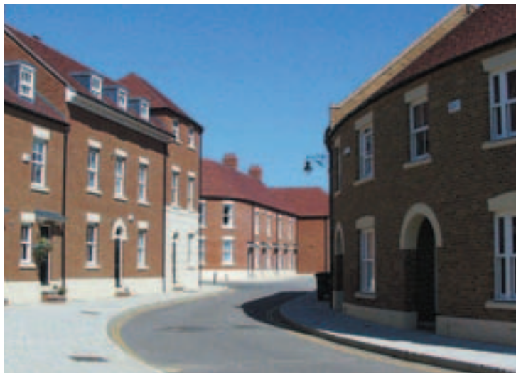
A combination of highway geometry and building line restrict forward visibility, reducing vehicle speeds. (St Dunstons Gate, Canterbury, Berkeley Homes)
