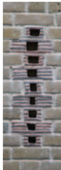
Air vents , close attention to material specification can lead to attractive and distinctive features instead of 'off the peg' solutions.
