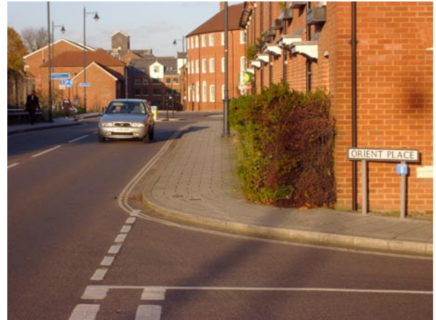
Examples of sight lines being achieved within necessary highway area, allowing for strong and flexible frontage treatment of properties.
