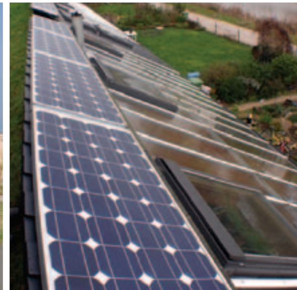
Solar or photovoltaic panels can provide a cost effective and environmentally responsible form of energy.
