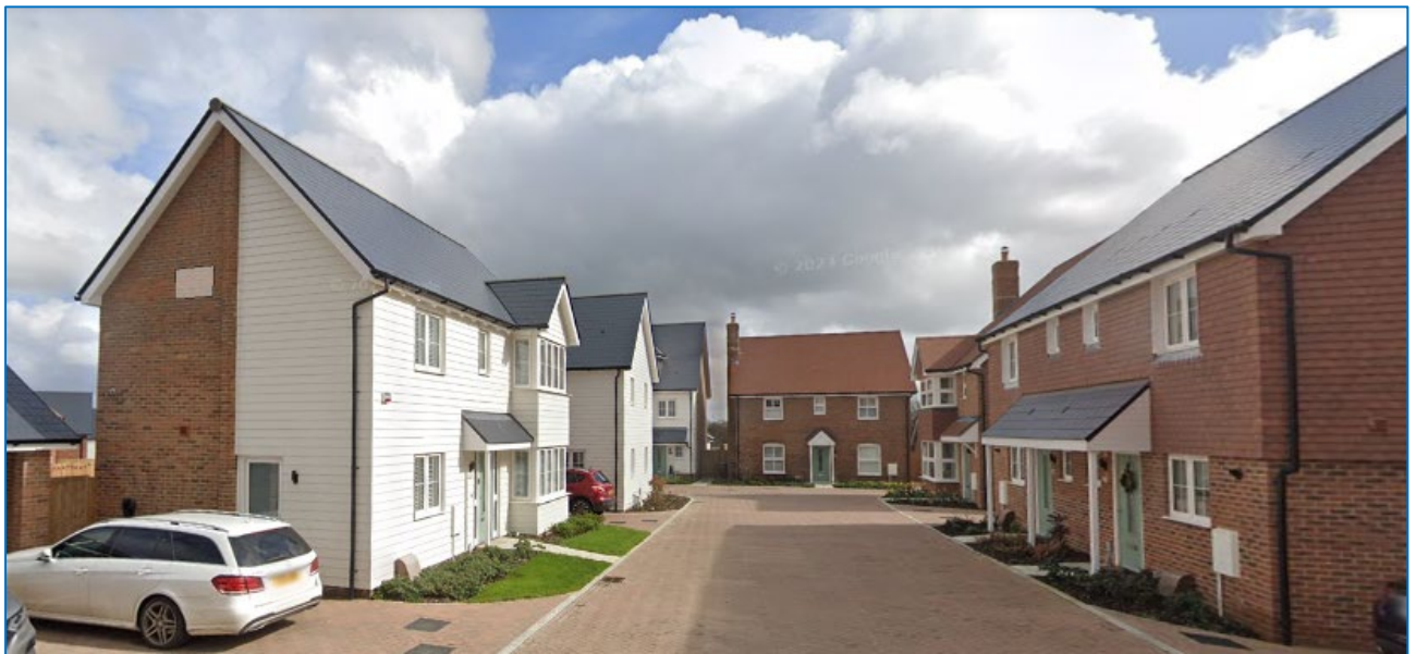
Figure 10: Kings Oak Park, Headcorn (site allocation H1(36)) (image: Google Maps, March 2023)
