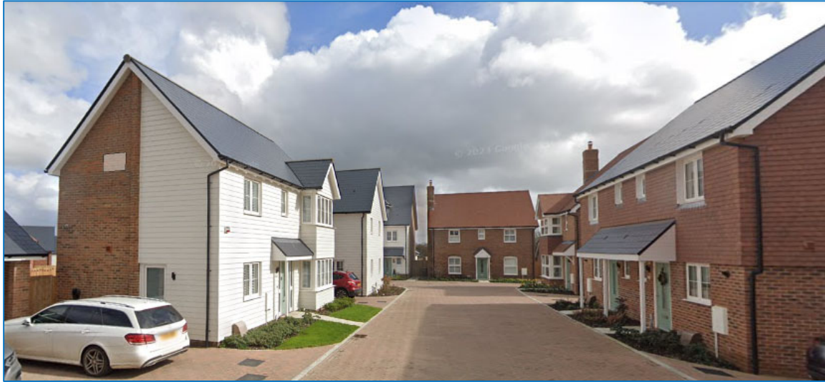
Figure 4: Kings Oak Park, Headcorn (site allocation H1(36)) (image: Google Maps, March 2023)
