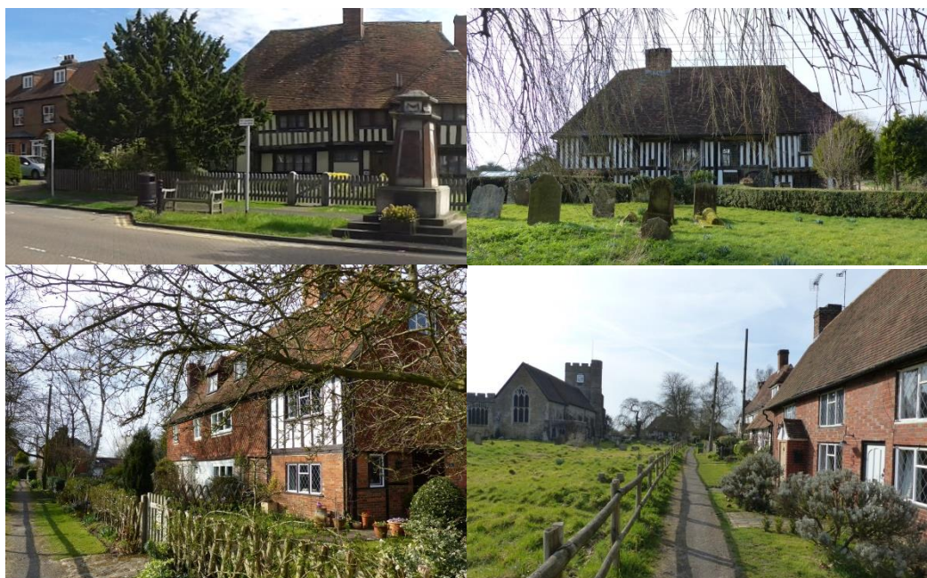
Figure 3: Examples of Headcorn's historic architecture
