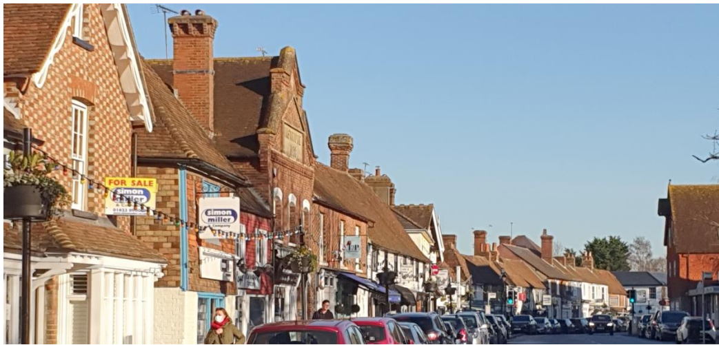
Figure 12: The roof line on the High Street
