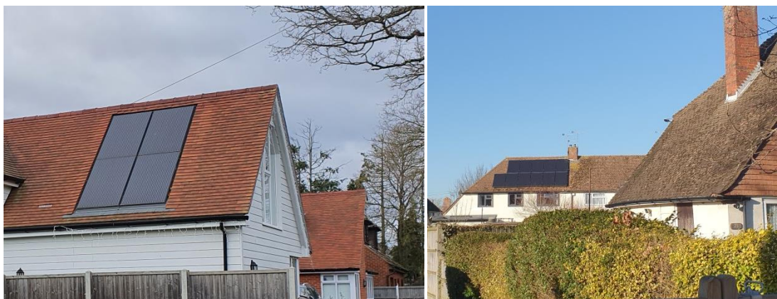
Figure 33: Integrating solar panels within roofs is visually more attractive than post construction bolt on options
