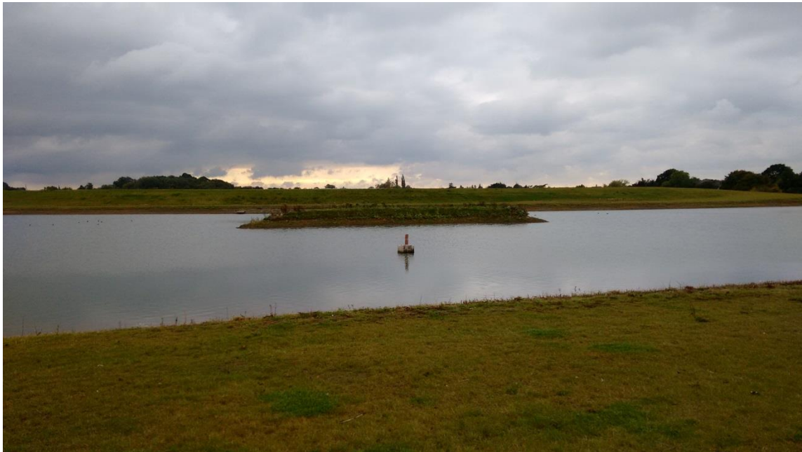
Figure A.9: View S over Lake 3, including outfall. Viewpoint 8.
