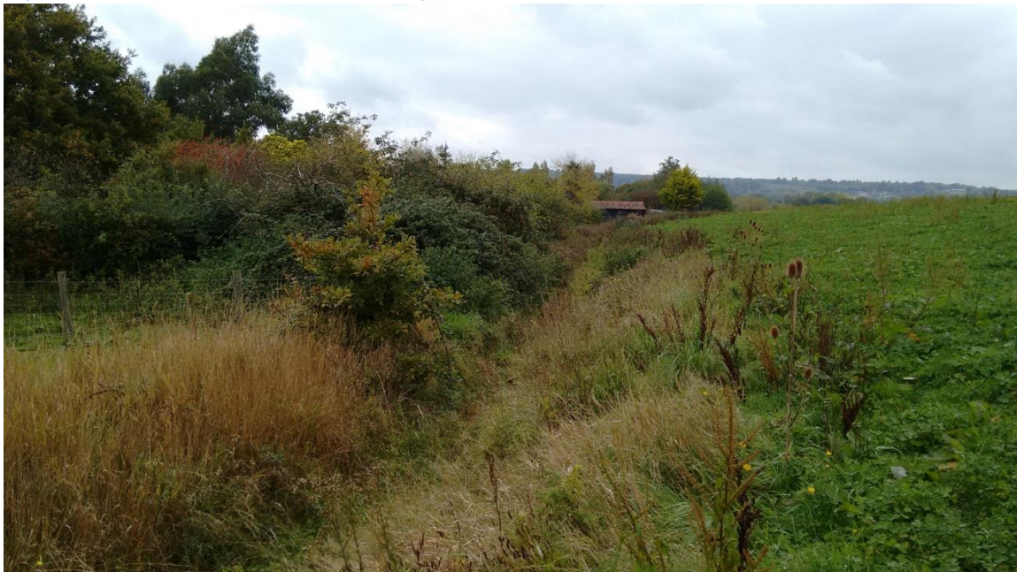
Figure A.5: Western boundary ditch looking NE from viewpoint 4 towards orchard
