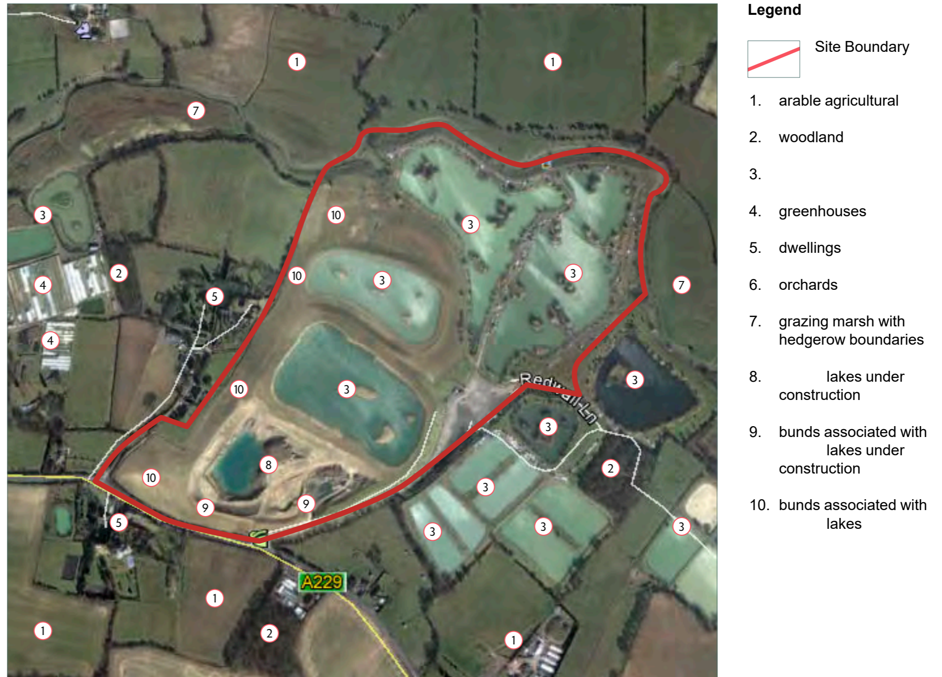
Figure 6.2 – 2014 aerial photography of Site (google earth - accessed Feb 2015)
