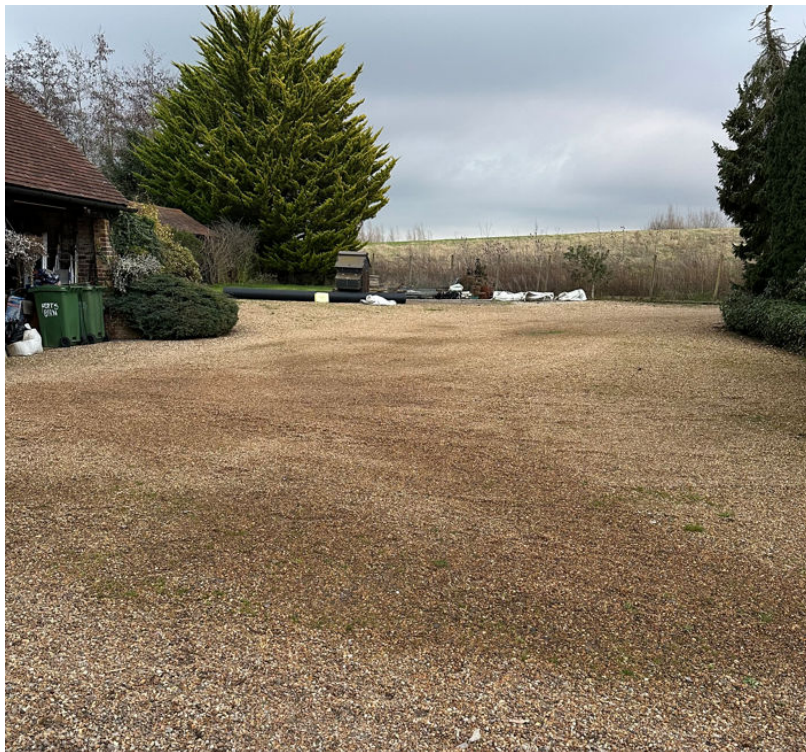
Water tracking across the driveway towards the house
