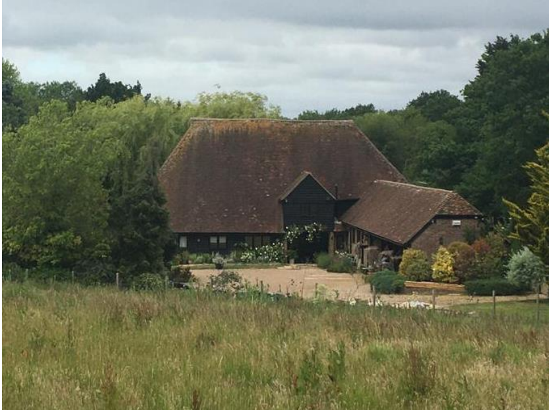
Figure 21: The eastern elevation of the Grade II Listed Barn when viewed from the Appeal Site as at June 2020 (NB. this view is zoomed in and should not be used to demonstrate the proportional distance)
