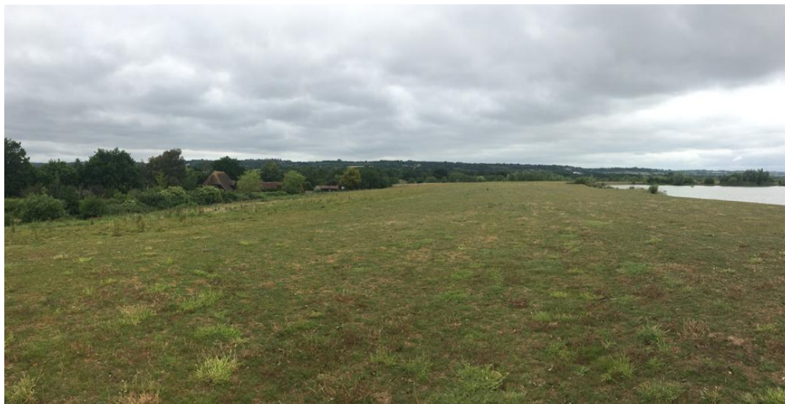
Figure 27: View from near Lake 1 looking north including Lake 2 and the Grade II Listed Barn depicting the shallow bank as at June 2020.
