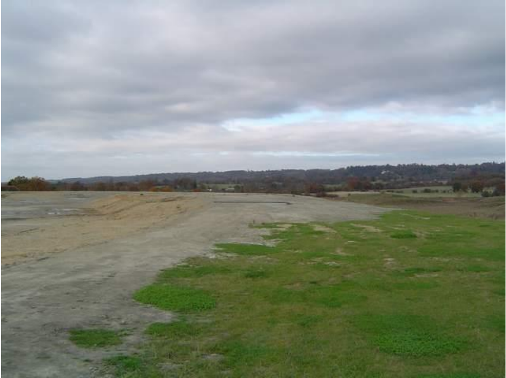
Crest near eastern corner looking north-westwards
