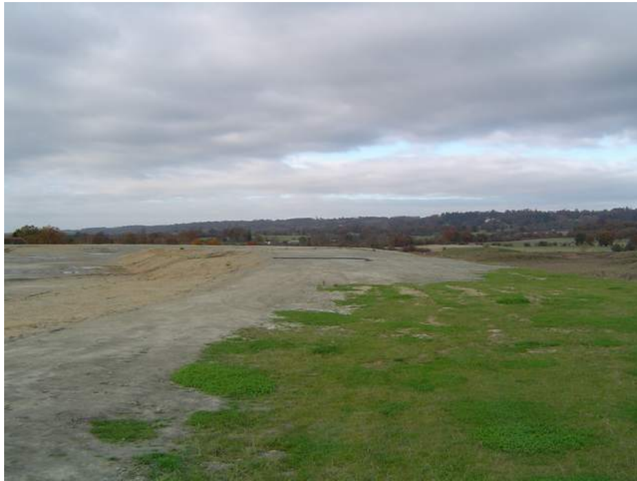
Crest near eastern corner looking north-westwards
