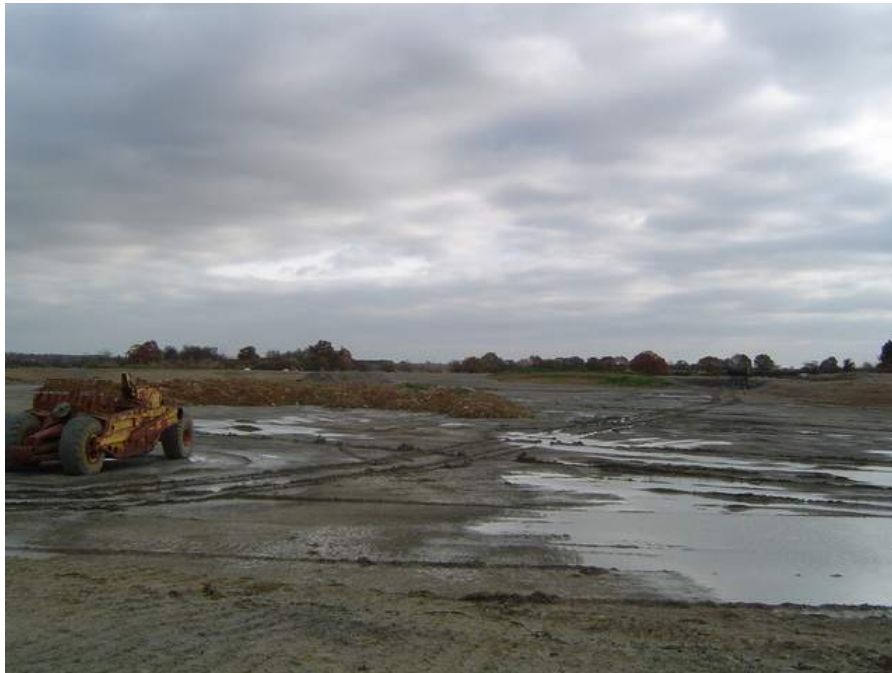
Internal floor of reservoir basin in the wetland area
