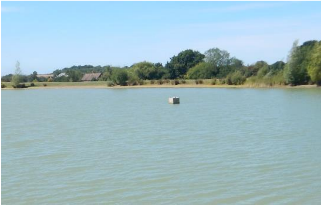
Photograph 11 Overflow viewed from embankment
