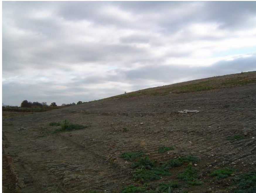
External slope at northern corner from embankment toe
