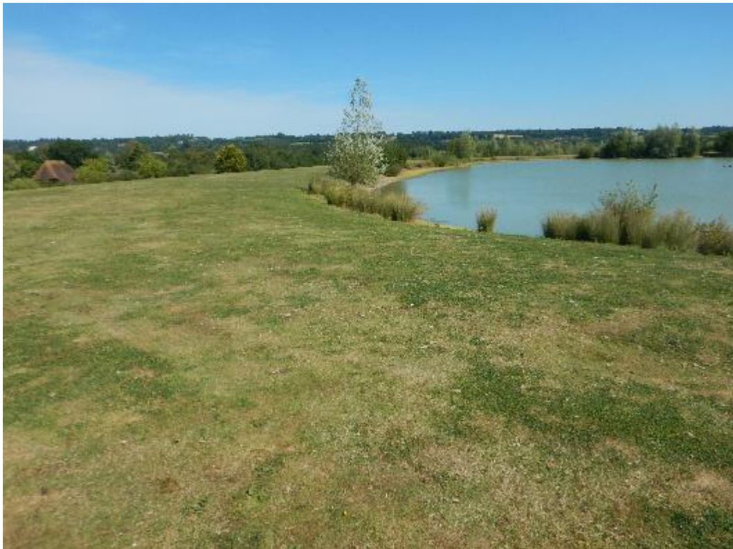
Photograph 6 West embankment crest and inner slope
