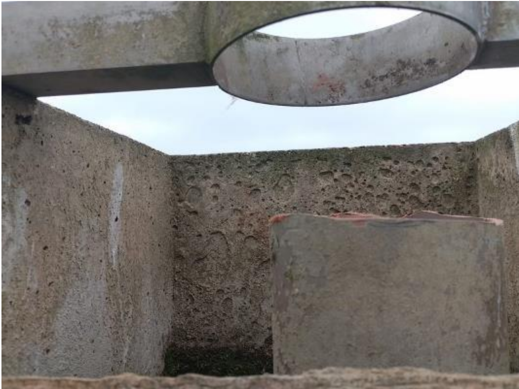
Photograph 13 Overflow pipe after cutting
