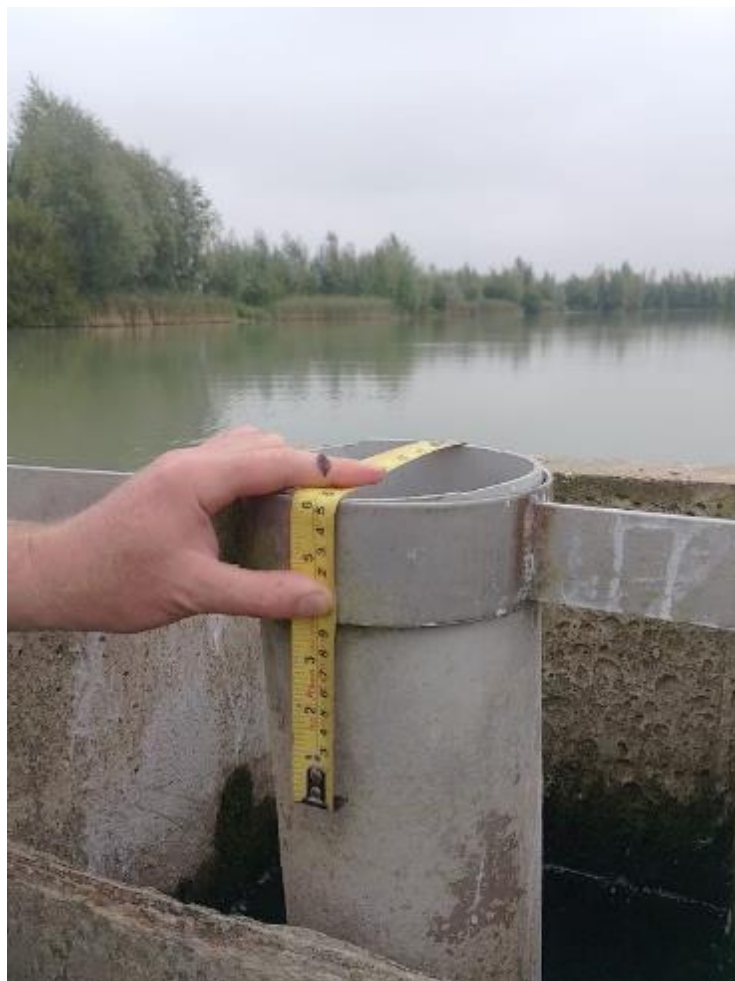
Photograph 12 Measuring overflow pipe before cutting 150 mm
