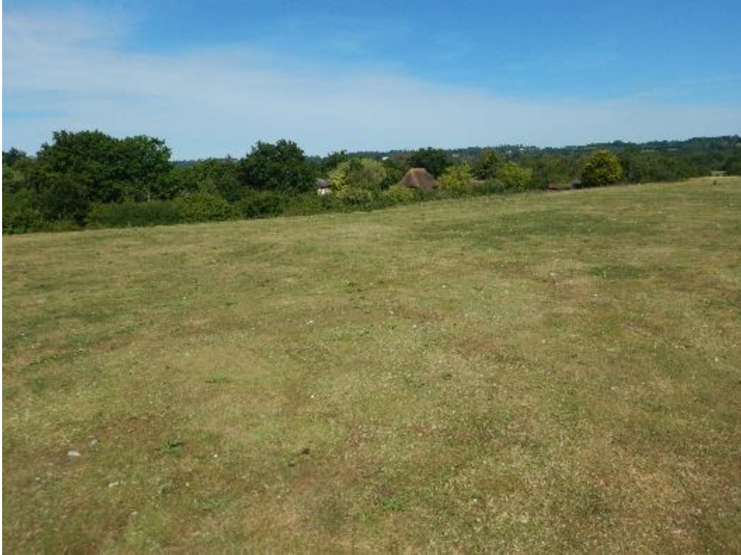
Photograph 7 West embankment outer slope
