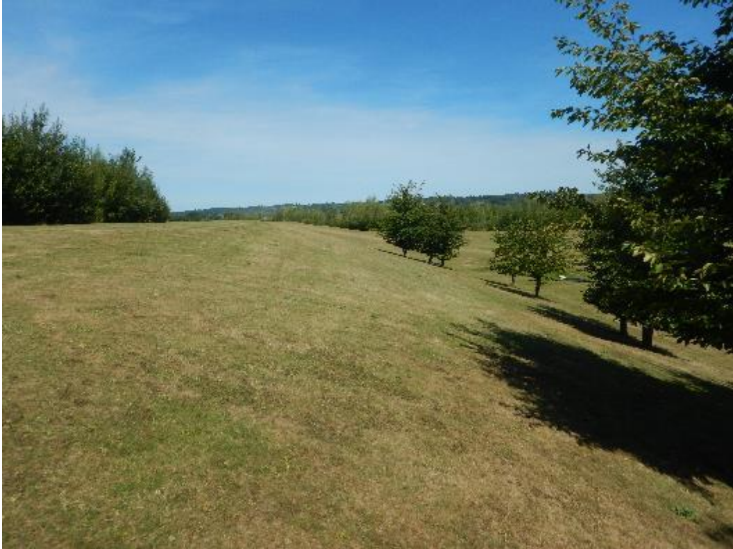
Photograph 1 East embankment outer slope
