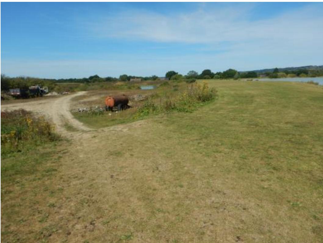
Photograph 4 South embankment outer slope
