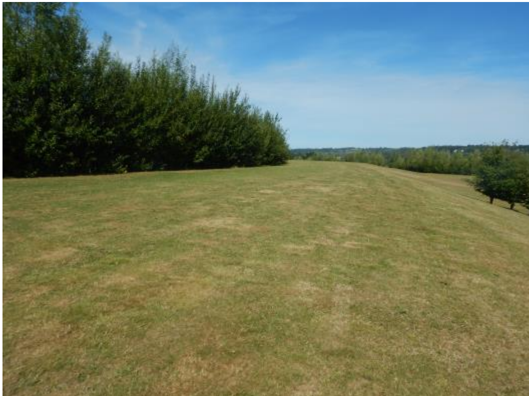
Photograph 2 East embankment crest
