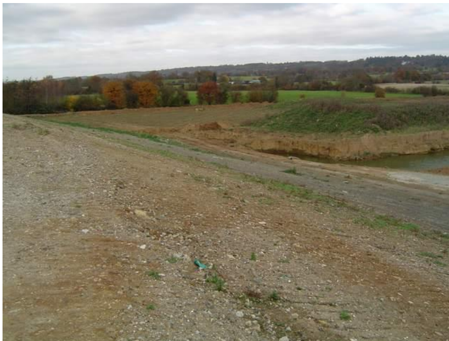
External slope at northern corner from embankment crest
