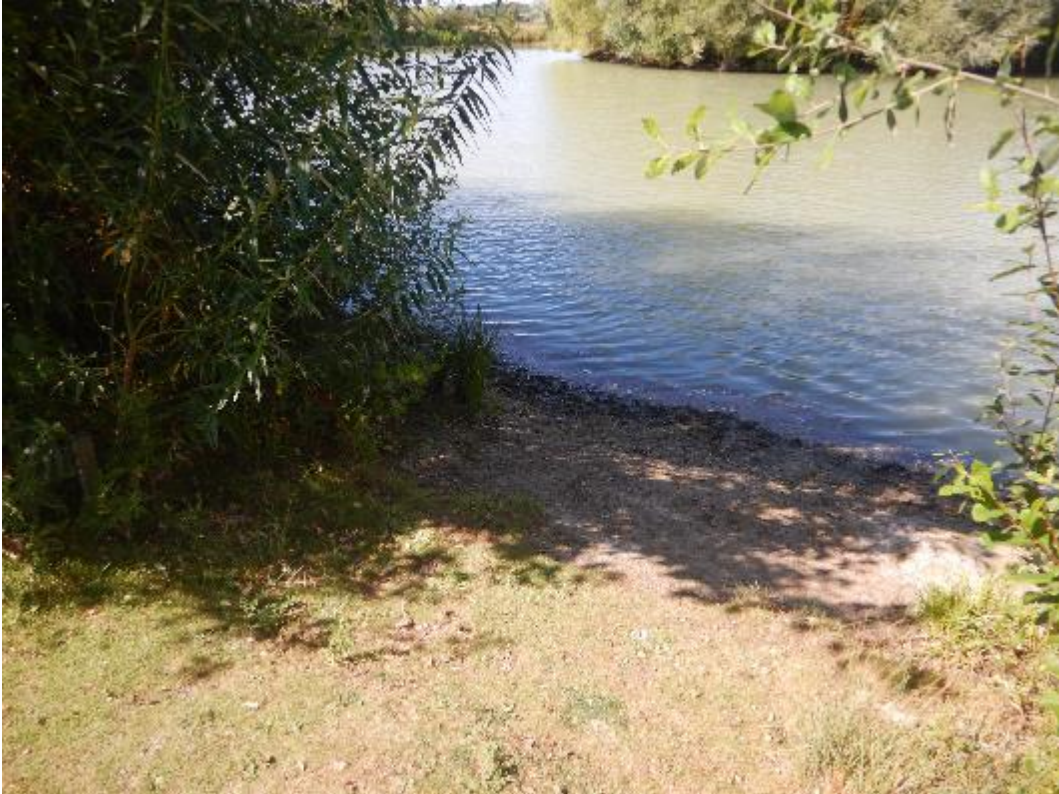
Photograph 3 East embankment inner slope
