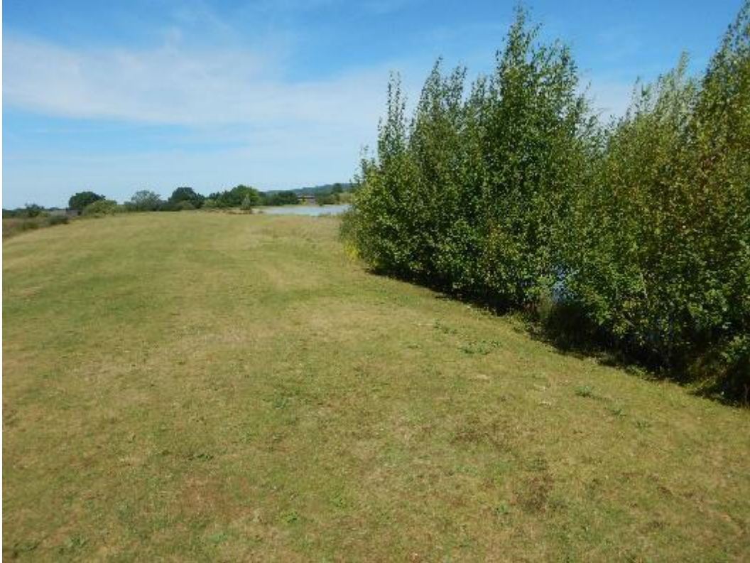
Photograph 5 South embankment crest and inner slope
