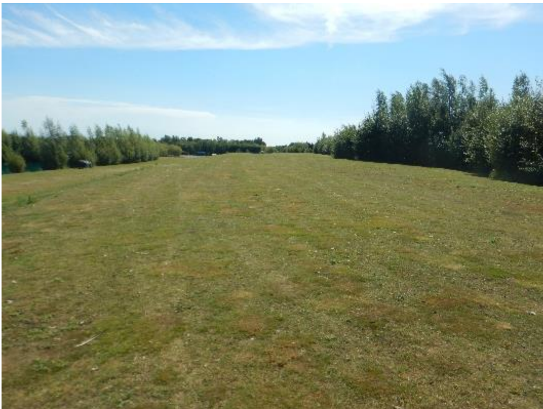
Photograph 10 North embankment crest
