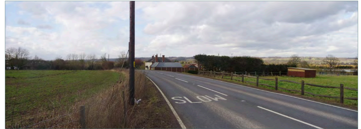
Photograph – Viewpoint 26 (February 2015) View looking northeast towards the appeal site from Staplehurst Road. From this elevated location partial views of part of the earthworks bund are evident through the intervening vegetation associated with Staplehurst Road.
