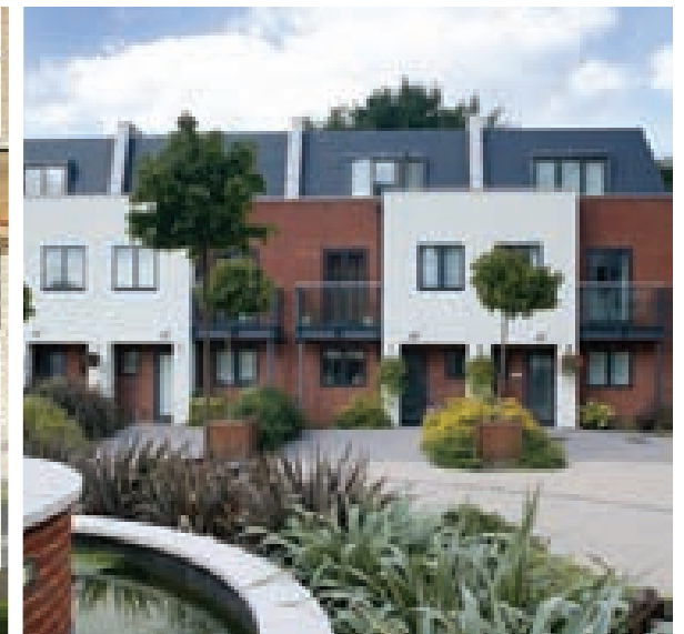
Versatile and adaptable homes can be provided by terraced housing. (Kings Gate, Horsham. Belmont Homes)
