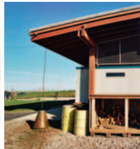
Romney Marsh visitor centre was built using a simple timber frame construction with straw bale infill with lime render and loose aggregate on floor and walls. Everything is either 100% salvageable or bio-degradable. (BBM for Shepway District Council)
