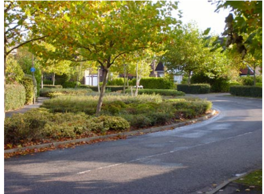
‘Old standard’ forward visibility curve which requires planting (except individual trees) to be maintained below reasonable growing height.
