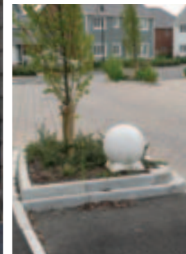
A simple feature built out to create a road narrowing will make drivers slow down. (Leybourne Lakes, Berkeley Homes)
