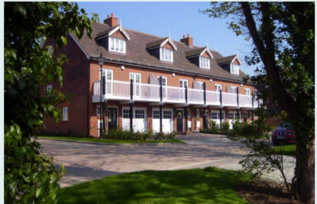
COLLEGE GARDENS, WESTGATE-ON-SEA Good materials and landscaping combine with quality design to achieve high levels of occupiers' satisfaction.
