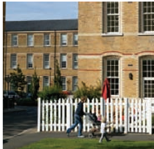
Reuse of buildings is sustainable and can lend a character that raises values in new development. (Caterham Barracks, by Linden Homes)
