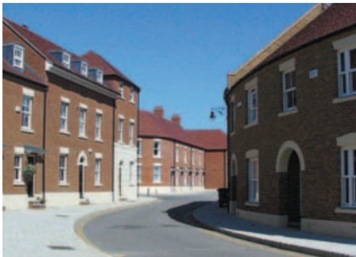
A combination of highway geometry and building line restrict forward visibility, reducing vehicle speeds. (St Dunstons Gate, Canterbury, Berkeley Homes)
