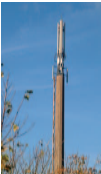
Masts can be designed to blend in with the surrounding landscape. This mast is clad in timber and sited within a heavily wooded area.
