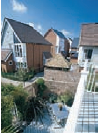
Overlooking without reducing privacy. Streets and spaces feel safe and secure when overlooked from homes and public spaces. (Lacuna, Kings Hill.)
