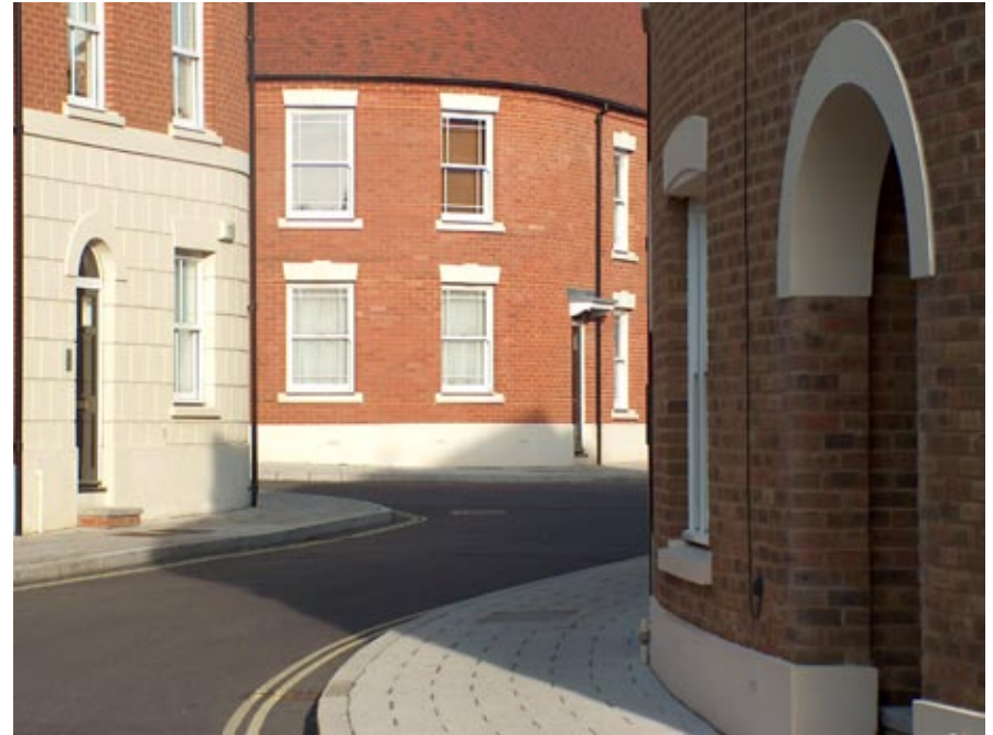
Acceptable forward visibility achieved without creating false building lines and/or widened footways.
